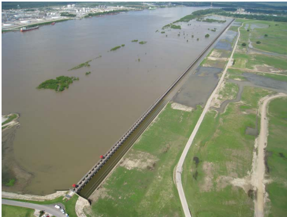
Figure 6. The Bonnet Carré spillway is a flood release valve along the low Mississippi River and discharges up to 28% of the flow of the river into the adjacent Lake Pontchartrain estuary (photo credit: Eddie Weeks).
