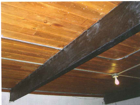
A retrofitted beam in the Coolidge Roundhouse Gymnasium is fully encased with a carbon-fiber covering
